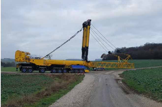
Figure 31: Site transport of a 750 tons Telescopic crane
