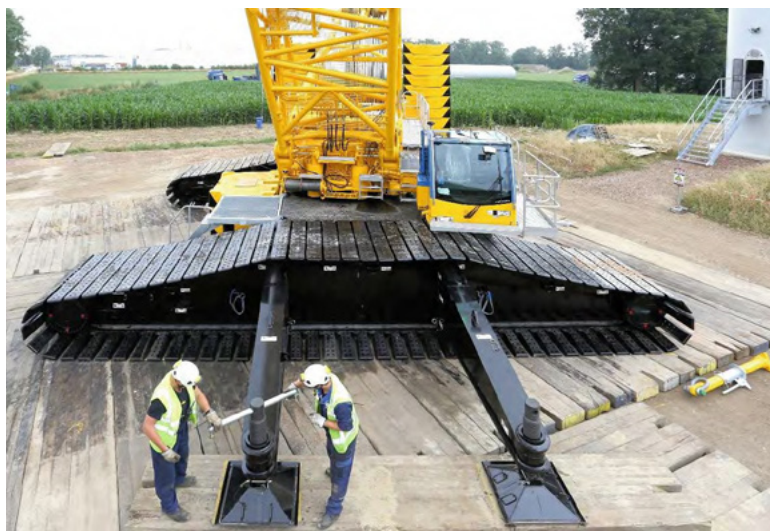
Figure 8: The up righting outriggers on a 600 tons crawler crane.
