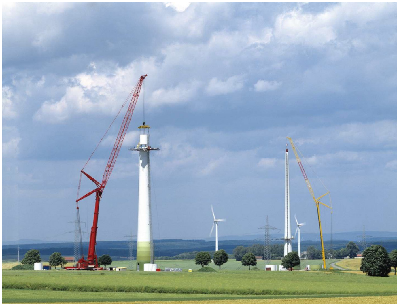
Figure 5: Two 500 tons hydraulic cranes equipped with luffing jib
