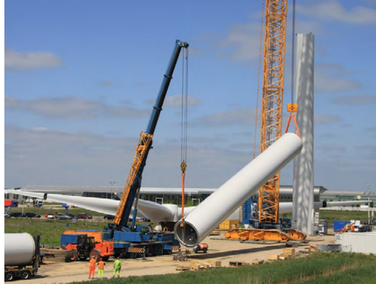
Figure 32: Example of a “tailing operation” with a main crane and a tailing crane
