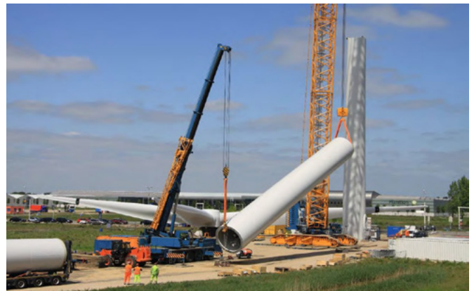
Figure 4: A tailing operation of a tower section
